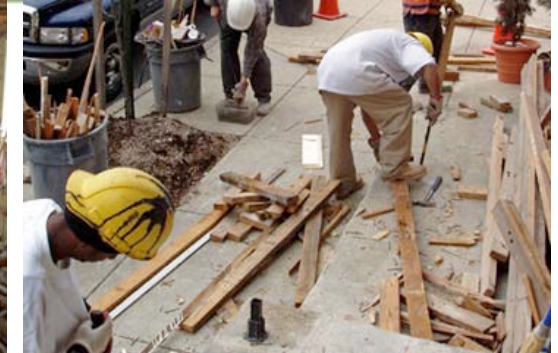
Pulling nails for recycling.
