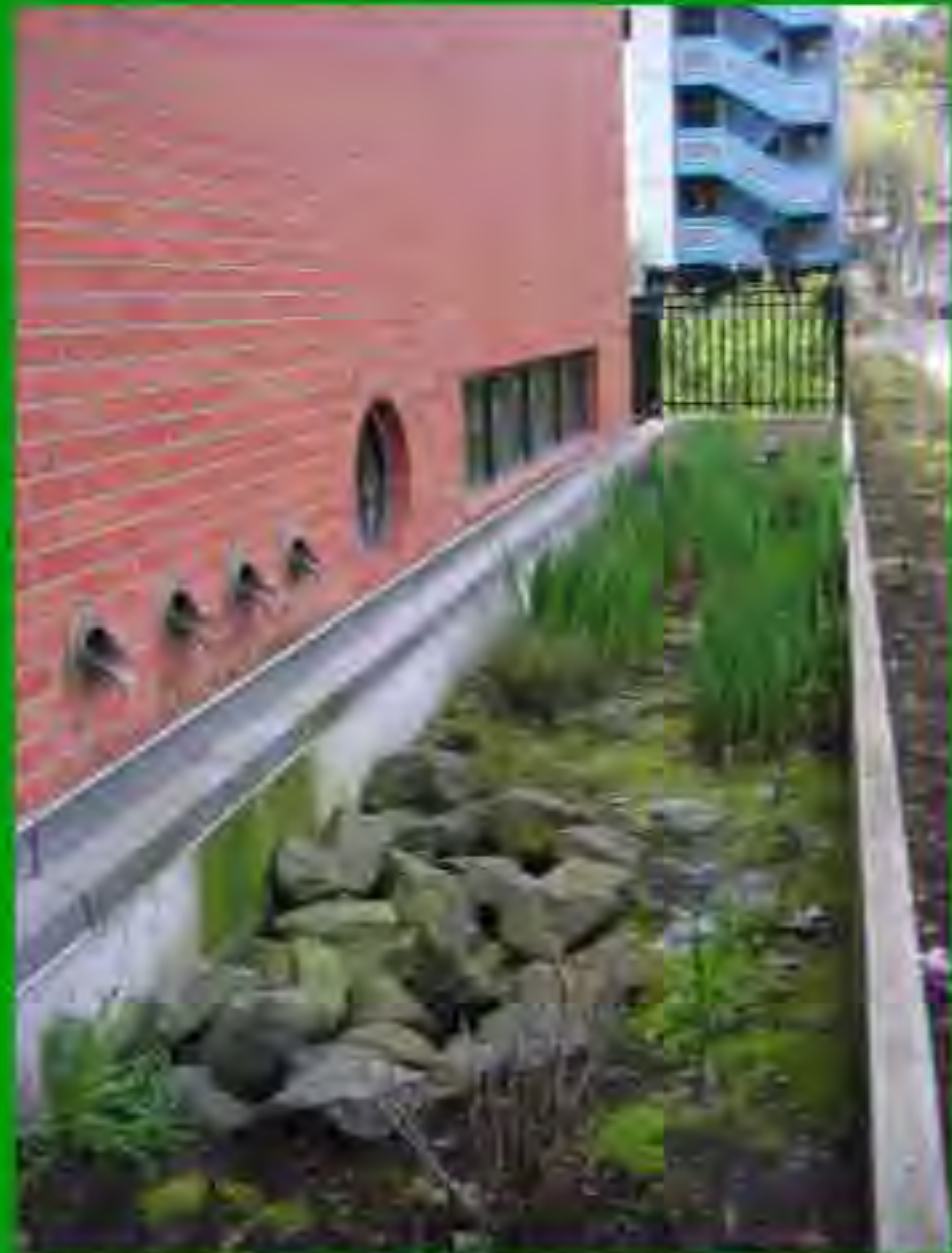
Vegetated Planter and disconnected downspouts at Portland State University. Photo courtesy of Martina Frey.
