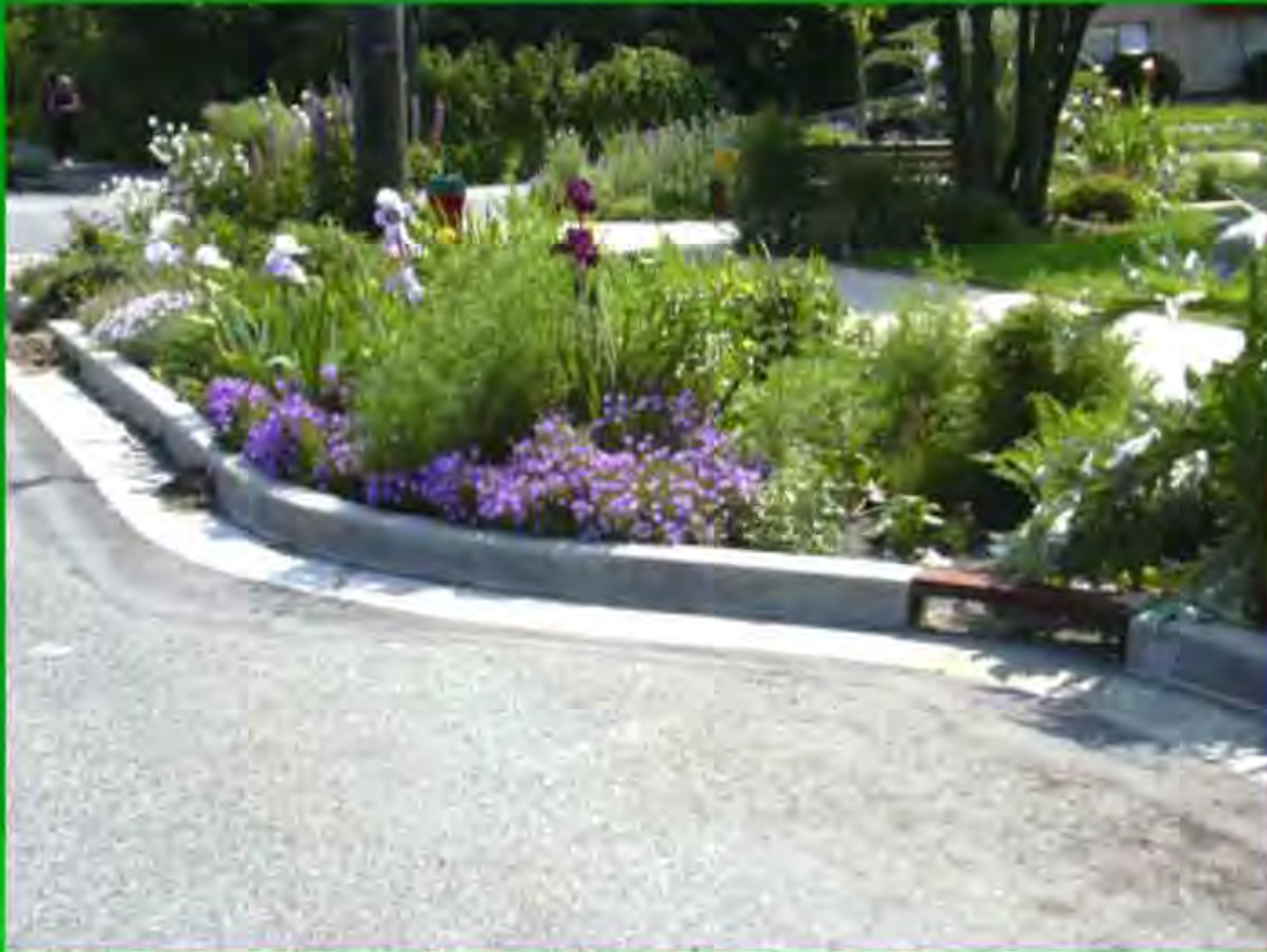
Infiltration bulge. Photo courtesy of City of Vancouver Greenways Program.
