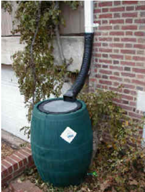
Residential rain barrels are an inexpensive and easy retrofit that reduces stormwater runoff and provides irrigation water. Photo at left: District of Columbia Water & Sewer Authority; Photo at right: Ann English.
