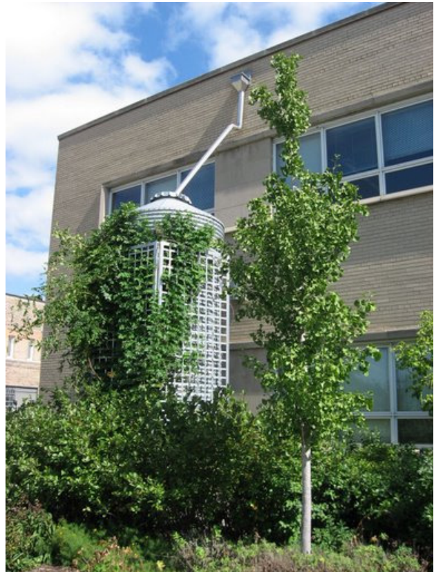
Commercially sized cistern at the Chicago Center for Green Technology. Photo: Abby Hall, EPA.
